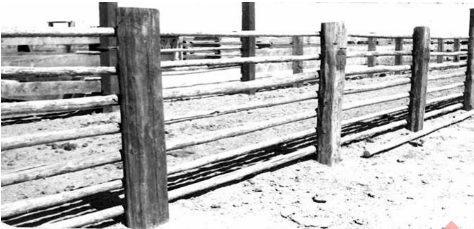
RAILROAD TIE POSTS 10' OC POLE RAIL FENCE AVERAGE QUALITY LESS 15 %
