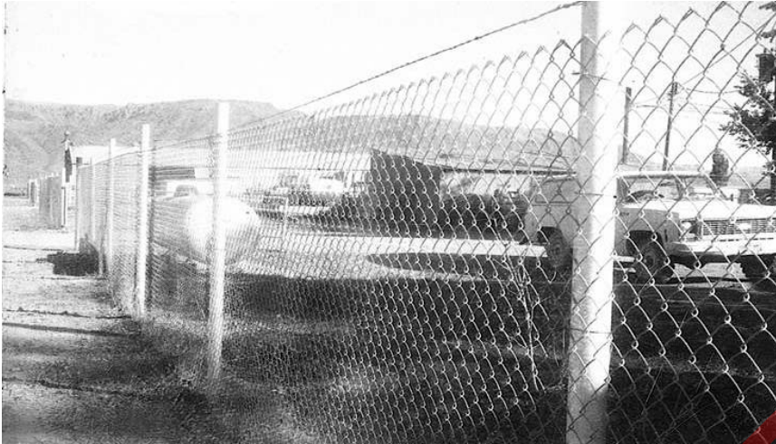
5' CHAIN LINK FENCE NO TOP RAIL
