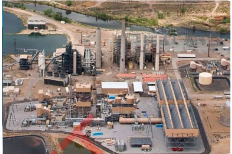
Nevada Energy's Tracy Power Plant (NV Energy Photo)
